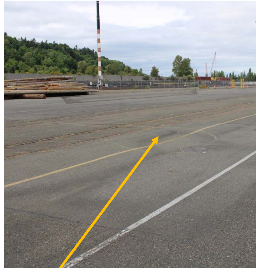
Subsidence at Manhole 2030
