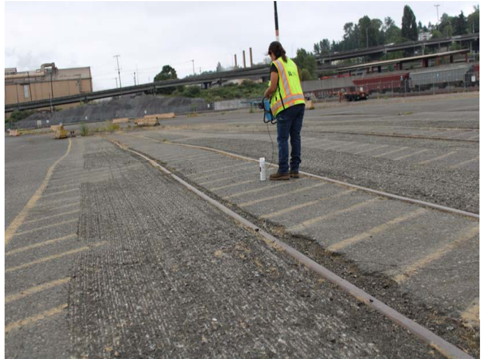
Surface and rail irregularities caused by slag
